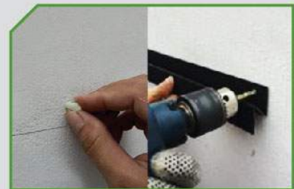
3. Insert the anchor bolts and screws into the holes to install the hanging bar.
